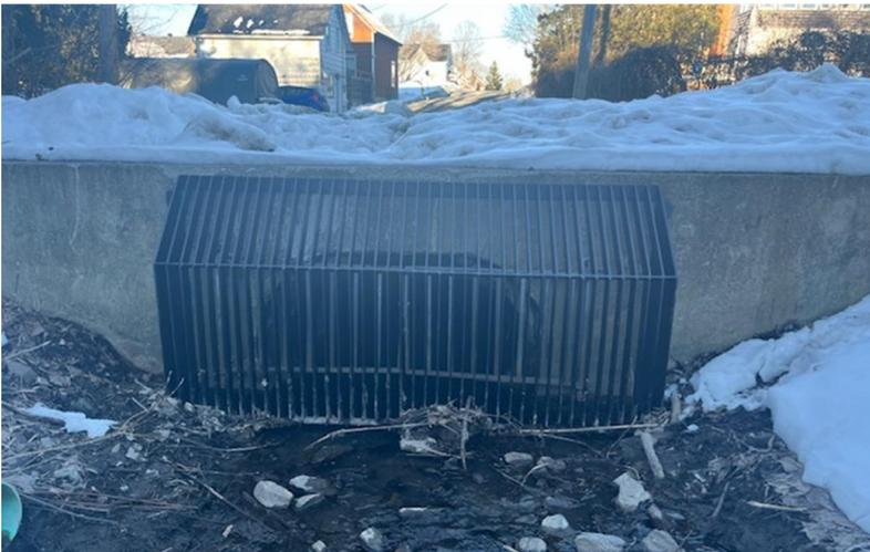
The Public Works Department is aware that during significant heavy rainfall events, there is the potential for flooding to occur at the corner of Lisgar Street and Argyle Street as there is a significant amount of water that flows to the headwall and then stormwater enters a pipe which then conveys the water to the Sussex Storm Pond. During
