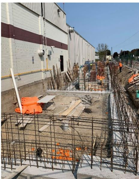
**September 22<sup>nd</sup>, 2020 Update** - Site fencing has been installed around the construction area and barricades set in place to create a temporary sidewalk adjacent to the work site. The area has been excavated and foundation work has commenced with footings poured last Friday. Foundation walls will be formed and poured this week. It is anticipated that masonry work will commence on October 1st, 2020.
