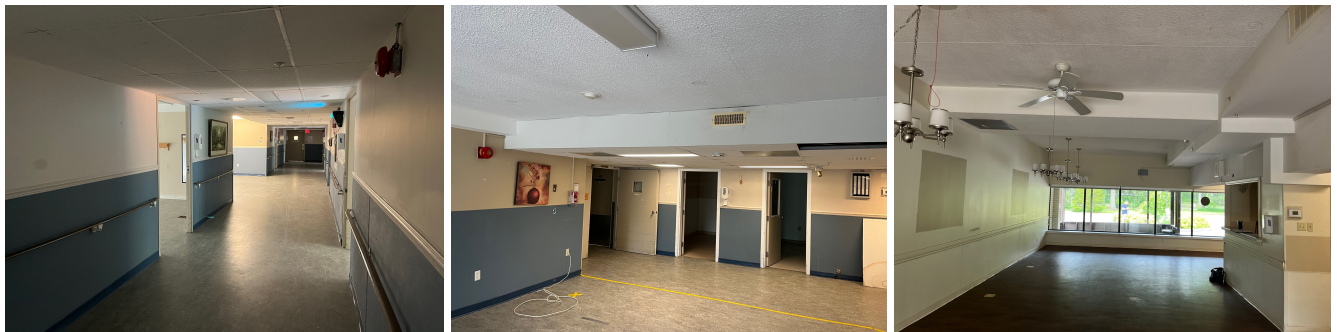
Photos 13, 14 & 15: Existing Interior Condition
