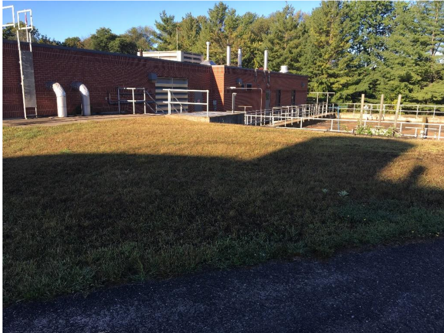
Photo 1: Existing structure and manicured lawn, facing southwest
