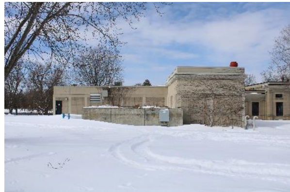
Plate 12: West elevation of contemporary addition
