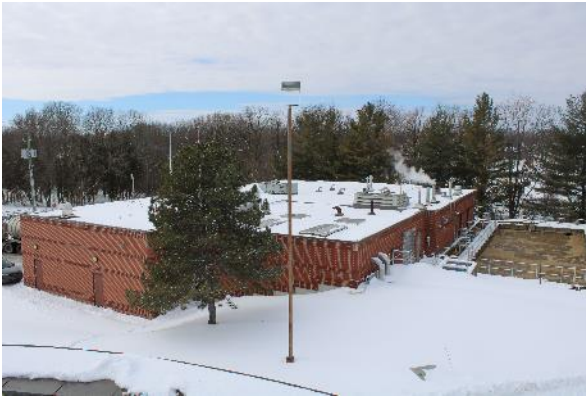
Plate 13: Main WWTP building from above
