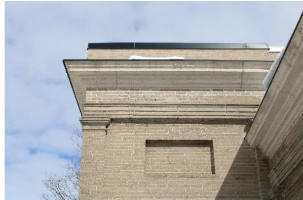
Plate 2: Detail of cornice and stonework
