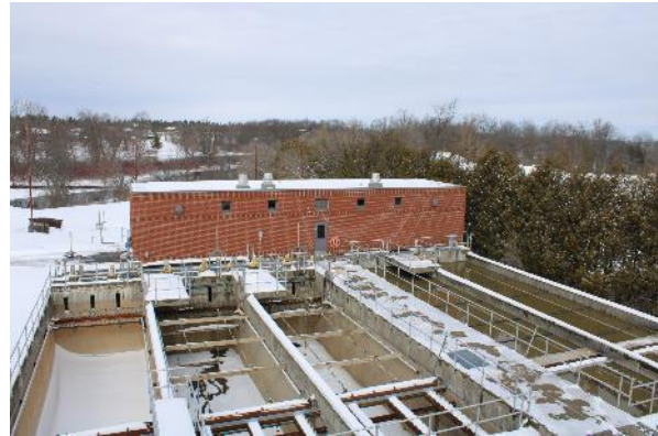
Plate 22: Aeration building and secondary tanks
