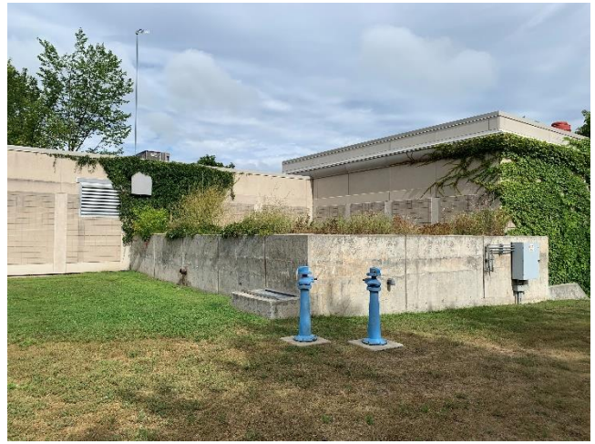
Photo 2: Site conditions of Water Treatment Plant (Site 1)
