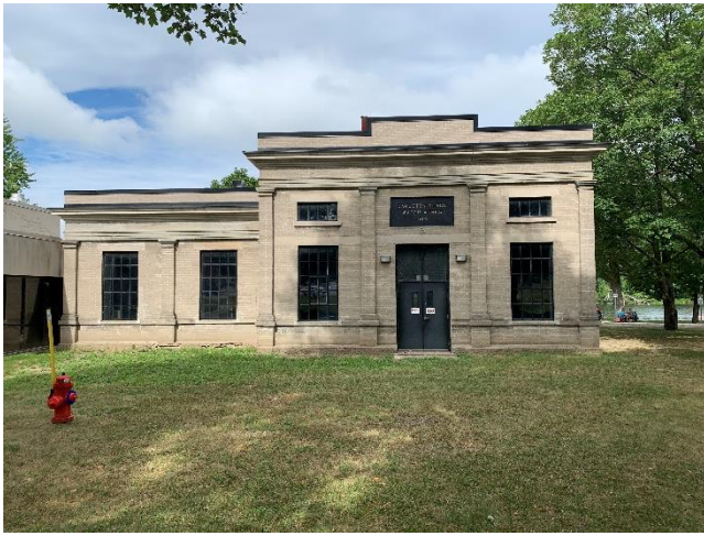
Photo 1: Site conditions of Water Treatment Plant (Site 1). Facing Northwest
