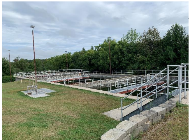
Photo 12: Site conditions of Site 3. Facing Northeast.
