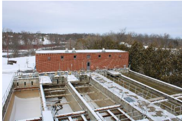
Plate 22: Aeration building and secondary tanks
