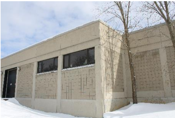
Plate 11: East elevation of contemporary addition
