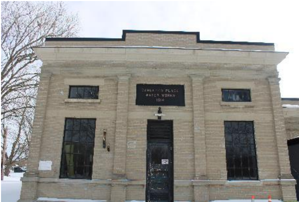
Plate 1: West elevation of WTP
