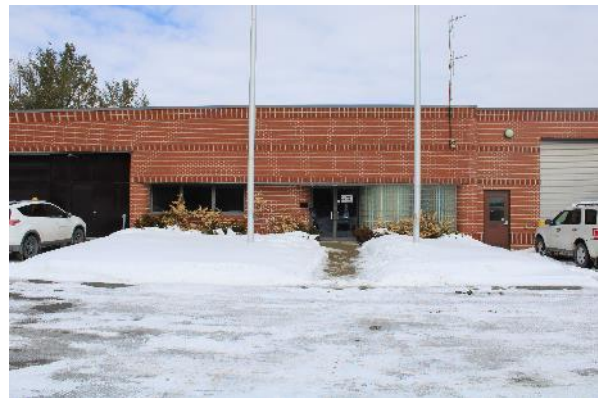
Plate 16: Entrance of main WWTP building
