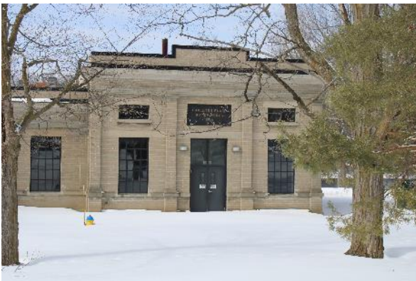
Plate 3: East Elevation of WTP
