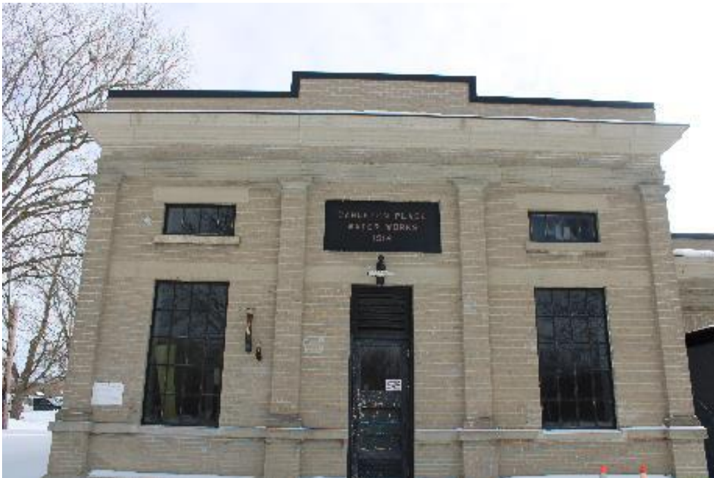
Figure 3.2: Photograph of Previously Identified or Potential Built Heritage Resource – 199 John Street – Carleton Place Waterworks (BHR-1)
