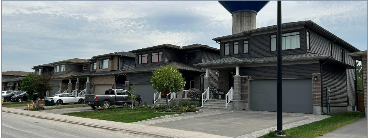
Figure 9: Existing Detached Dwelling Units on Christie Street (Source: Cavanagh Developments)
